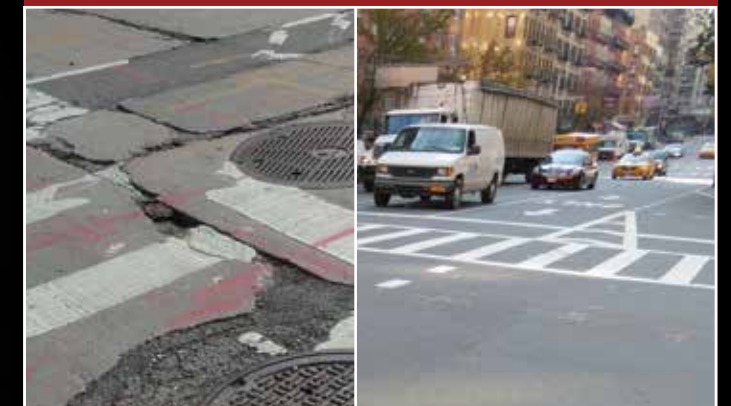
NYC's 1st Avenue – before and four years after application of FlexGard® and StellarFlex® HiMA
